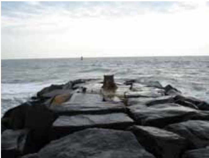
All that remains of the jetty tower is it's concrete base.
